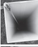
**10.** Screw the threaded rod snugly into the coupling nut at the bottom of the column and tighten with pliers.
