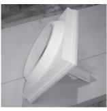
**11-12.** Locate the column cap shown in photos 11 and 12. Place on the column and feed the threaded rod through the hole in the center of the plate with the welded angle.
