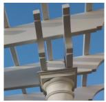
**11-12.** Locate the column cap shown in photos 11 and 12. Place on the column and feed the threaded rod through the hole in the center of the plate with the welded angle.
