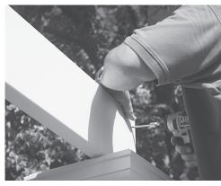
14. Install the rafter supports (will have "L" brackets installed to tops of supports) with the decorative rafter tails to the outside of the plate flanges using 2.5" hex head stainless steel self-tapping screws. Set clutch on the drill so the screw is not stripped.
