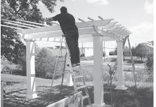
**19.** Set the clutch on the drill to ensure that the screw head does not dimple the top surface of the purlin. Continue across the top of the rafters until all purlins have been installed.
