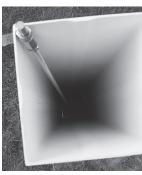
**10.** Screw the threaded rod snugly into the coupling nut at the bottom of the column and tighten with pliers.
