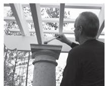
**20.** Using a 15/16" deep well ratchet or open end wrench tighten the nut on top of each column until very tight.
