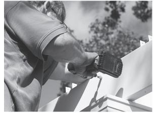
**15.** Install the rafter supports with the decorative rafter tails on the outside of the other aluminum angle using 2.5" hex head stainless steel self-tapping screws. Set clutch on the drill so the screw is not stripped.
